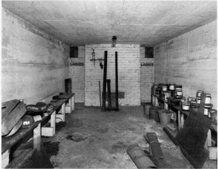
The ladies day room with two chemical toilet recesses and an emergency exit shaft at the far end.
